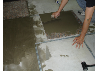
apply adhesives on tiles
