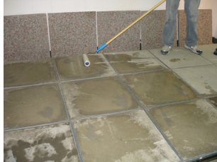
rinse panels and tiles
