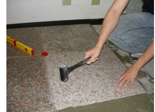
insert tile spacers, form 2 mm gap for grouting, check leveling
