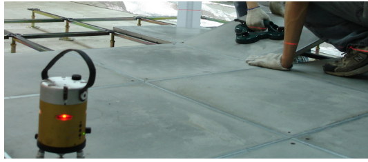
Install access panel and check level in sequence
