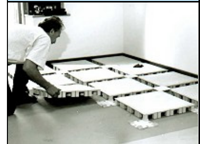
Connect by Base Connector. Installation is easy and fast.
