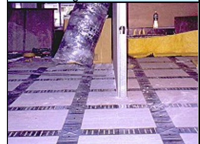
Internal dry wall or de-mountable partition can be installed on top of Netfloors.
