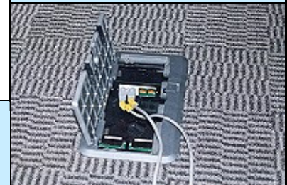
4. service box SB-603 installed at Cable Trench.
