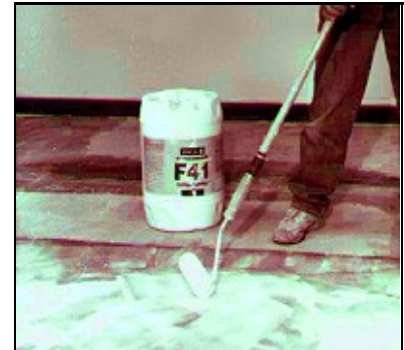
Apply adhesives at the Sub-floor by long-hand paint roller. Apply Sound Attenuation Blanket.
