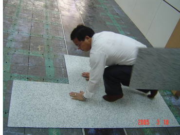
Install Actile on access (OA) floor same procedure as PVC tile.
