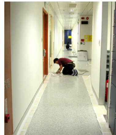
retrofitting on old HPL access floor, using double-side tape.
