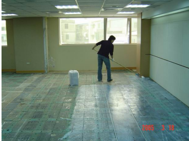
Remove old carpet tiles. Brushing releasable adhesive.
