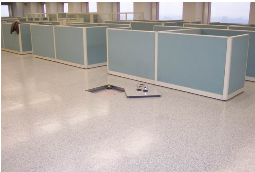
Actile one-to-one alignment bonding at the access floor panel without trimmer.
